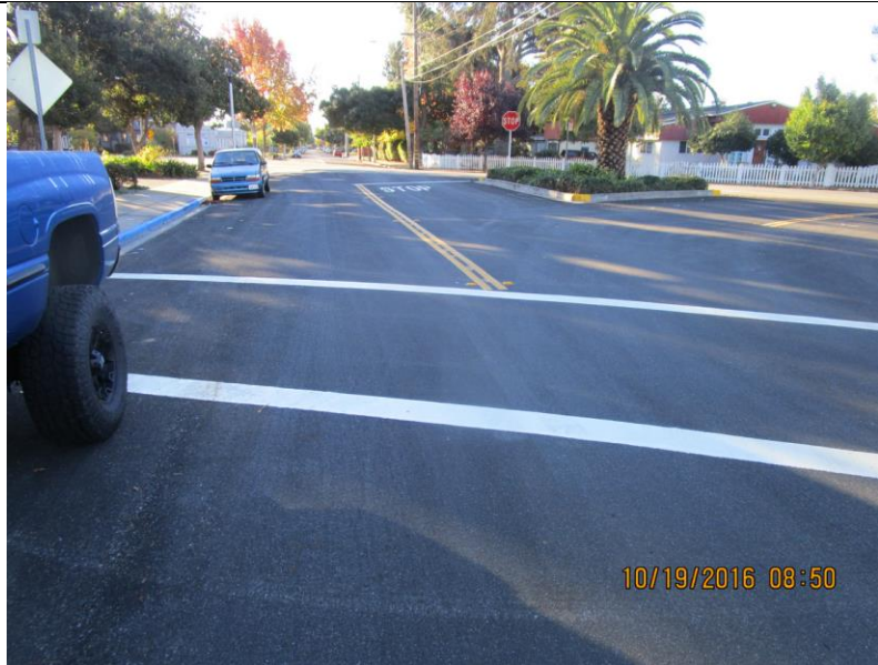
COMPLETED SLURRY SEAL ON BREED AVENUE
