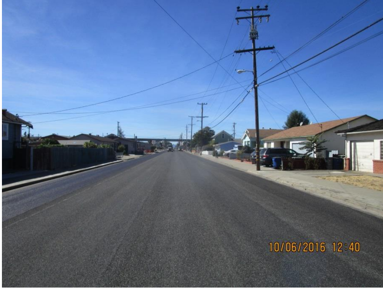
COMPLETED CAPE SEAL ON WILLIAMS STREET
